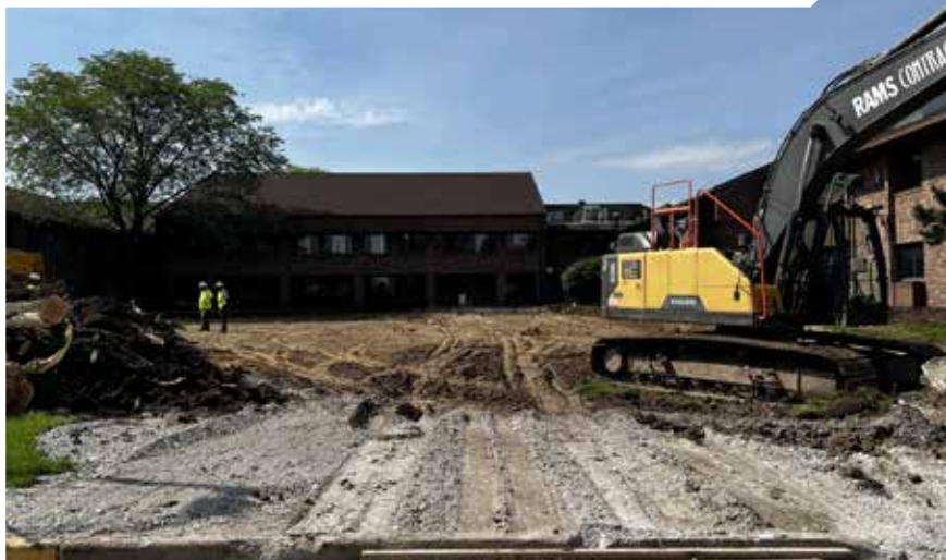
THE NEW COURTYARDS ENTRANCE UNDER CONSTRUCTION
